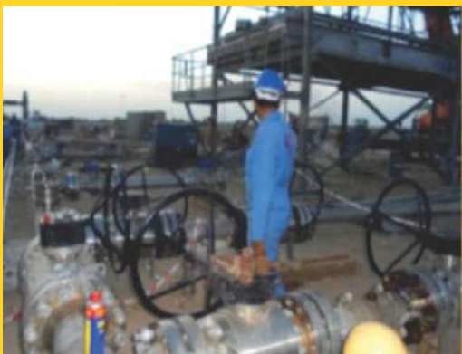
▶ Erection of Piping
