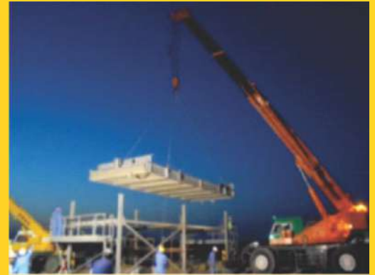
▶ Erection of Wellhead Cooler
