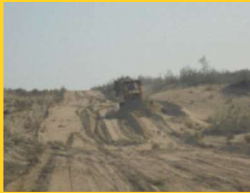
▶ Flowline ROW Grading
