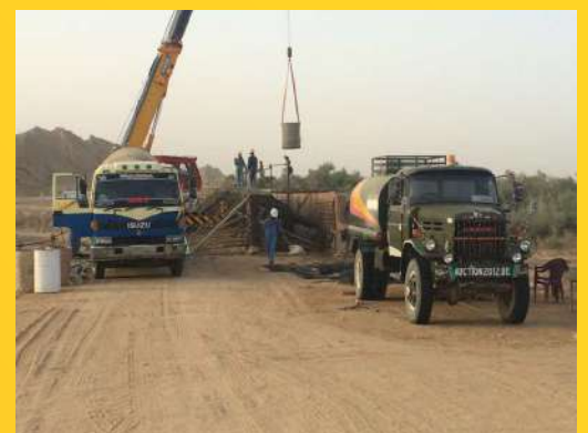
▶ Concrete of Bridge Girder
