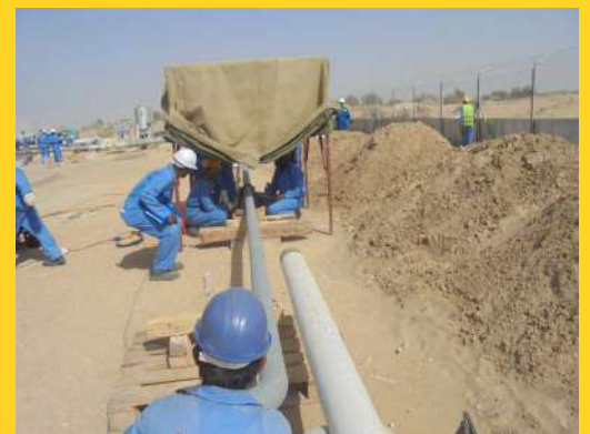
▶ Fabrication of CS Piping
