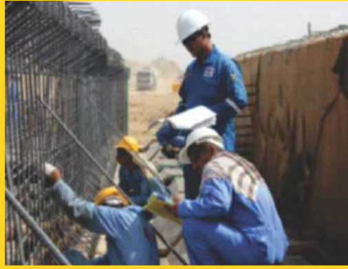
▶ Steel Fixing of Pre-Stress Girder
