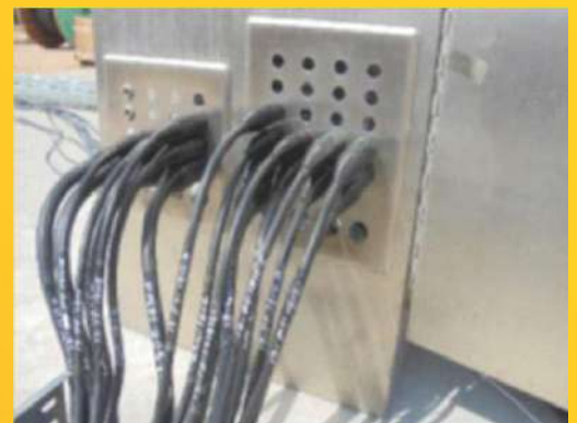
▶ Installation of Instrument Cables
