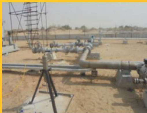
▶ Erection of Sample Bottle
