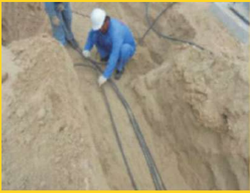
▶ Dressing of Cables in Trench
