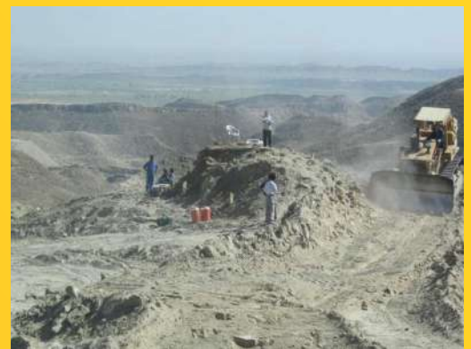
▶ Cutting of Rock for Road Works
