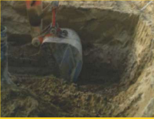
▶ Excavation for Celler Pad
