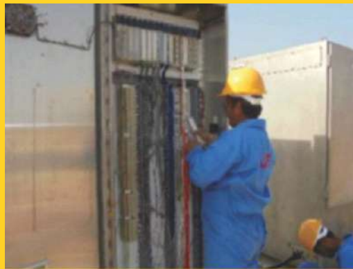
▶ Termination of Cables in Control Panel
