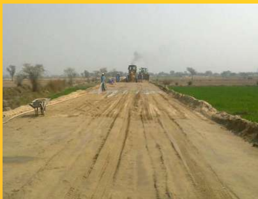
▶ Construction of Rig Road
