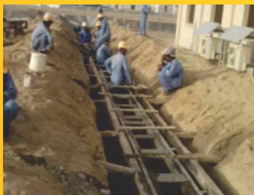
▶ Concrete of Internal Drain
