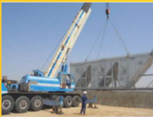
▶ Erection of Compressor Cooler
