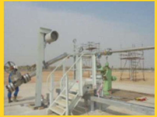
▶ Erection of Steel Structure
