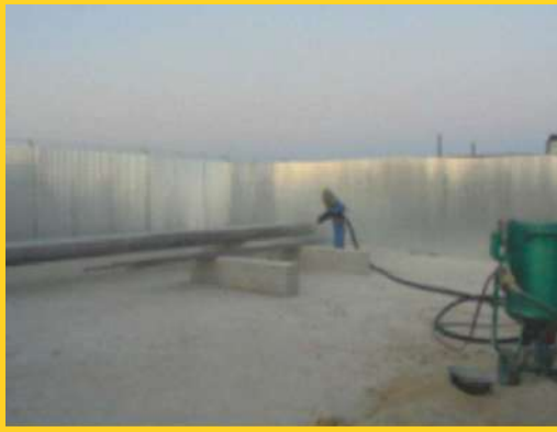
▶ Sand Blasting of CS Piping
