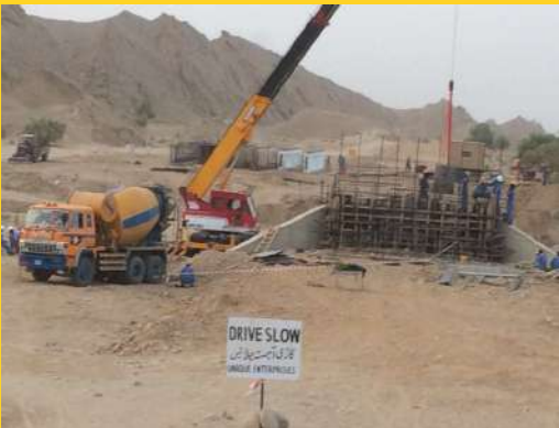
▶ Concrete for Bridge
