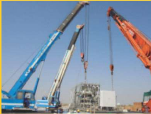
▶ Erection of wellhead Compressor
