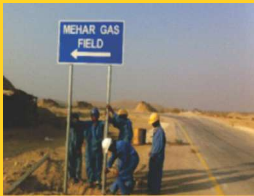
▶ Installation of Road Signs
