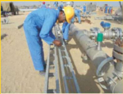
▶ Installation of Cable Tray
