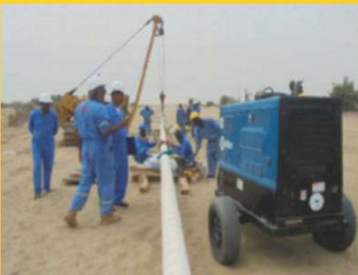
▶ Fabrication of Flowline
