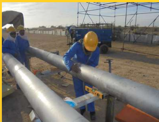
▶ Fabrication of Duplex Piping
