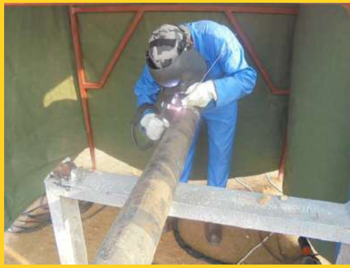
▶ Duplex Piping Welding
