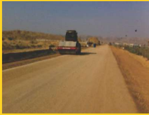
▶ Compaction of External Roads
