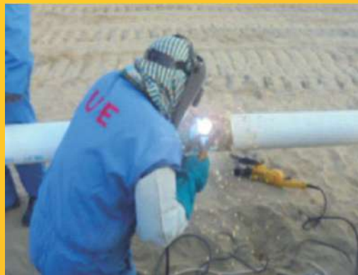
▶ Welding of Flowline
