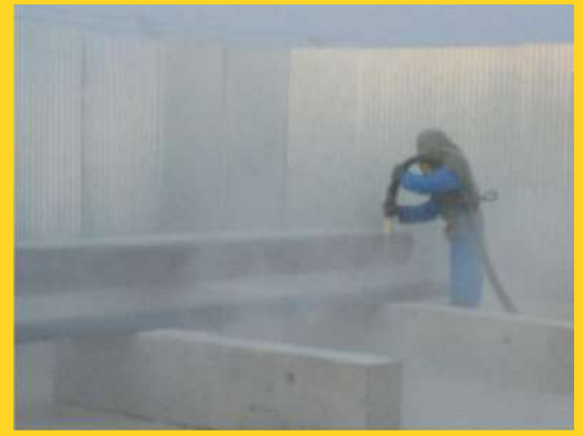
▶ Sand Blasting of CS Piping
