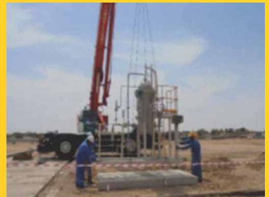
▶ Erection of Sour Gas Skid
