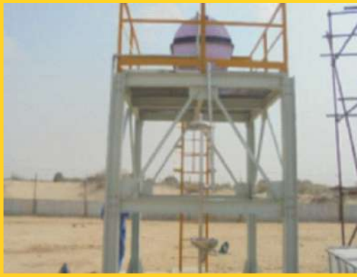
▶ Fabrication & Erection of Eye Wash Shower
