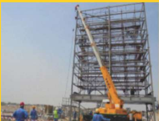
▶ Erection of Cooler Structure
