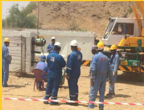
▶ Pre-Stressing of Bridge Girder
