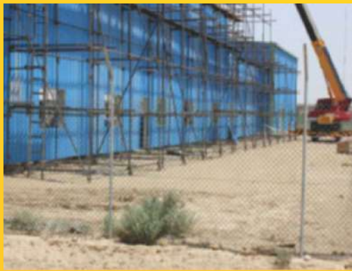
▶ Fabrication & Erection of Sheds
