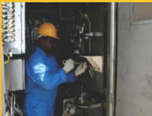
▶ Erection Hydraulic Pannel
