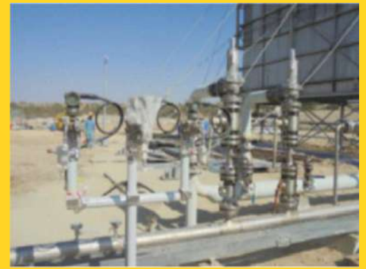
▶ Installation of PSVs
