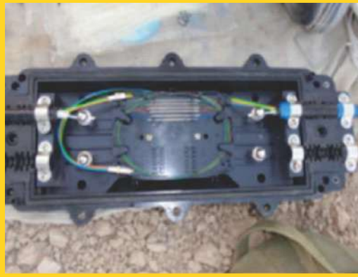
▶ FOC splicing & Jointing
