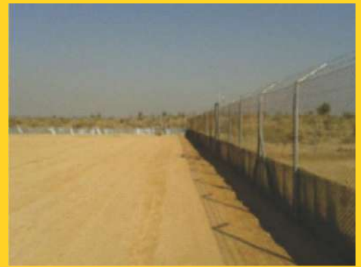
▶ Fabrication & Installation of Fence
