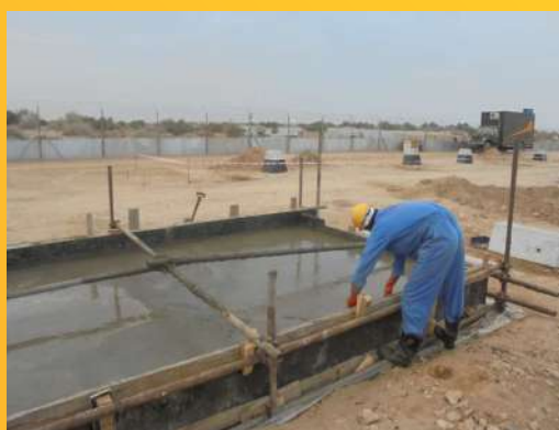
▶ C.I Skid Foundation
